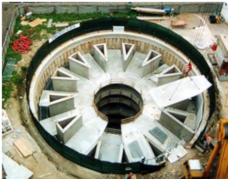
Fig 4: Birds-eye view of construction of Perfect Park
