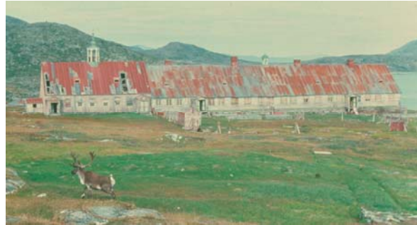
The abandoned Moravian mission building at Hebron, 1978. Photo: Steven Cox, Torngat Archaeological Project.
