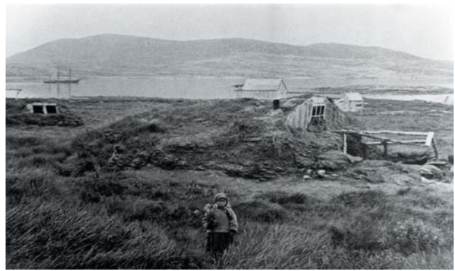
Inuit house at Hebron ca. 1910. Sod-covered wooden-frame cabin combines traditional Inuit house construction elements (sod-walls for insulation, south-facing window, and porch configuration) with introduced European influences (wooden walls and wood-burning stoves). Photo: Samuel King Hutton , Among the Eskimos of Labrador , 1912.
